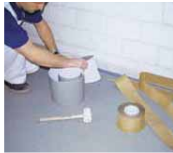
Formation of skirting with noraplan ® rubber floor covering
